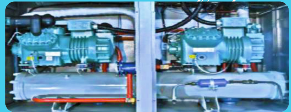
Compressor with Cascade Design
